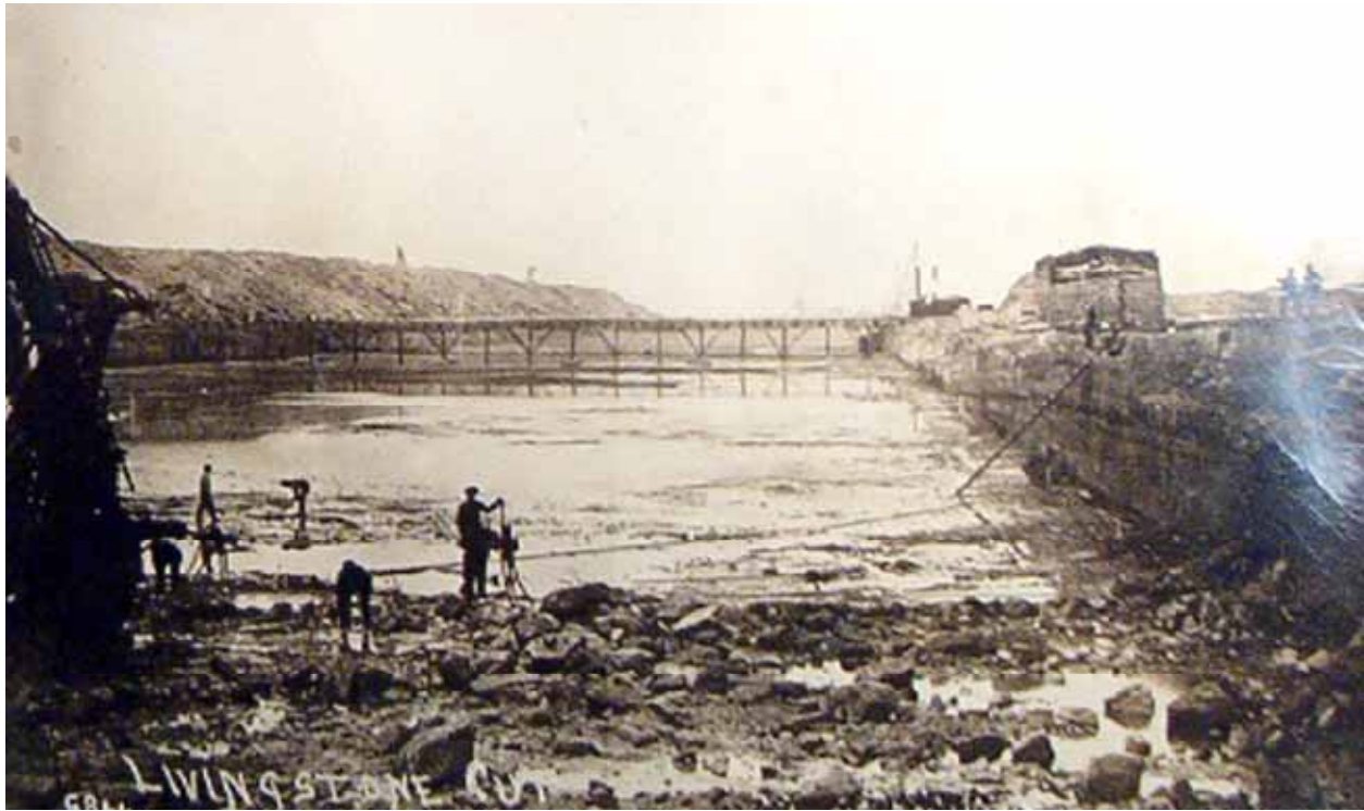
Figure 6. The Livingston Cut under construction in the Detroit River ca. 1910.
